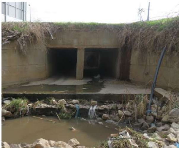
Drainage channel outlet discharging industrial effluent to the stream. Photo: Segev Tamir, Moran Development and Consulting
